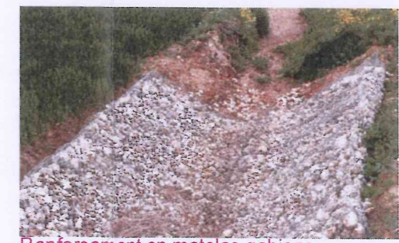
Renforcement en matelas gabions
