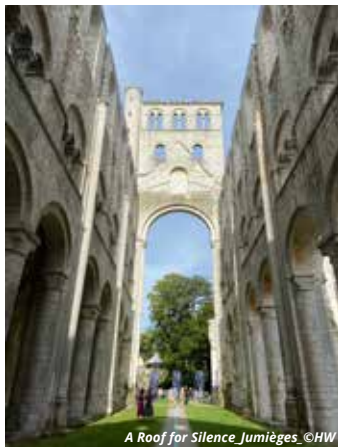
A Roof for Silence Jumièges ©HW
